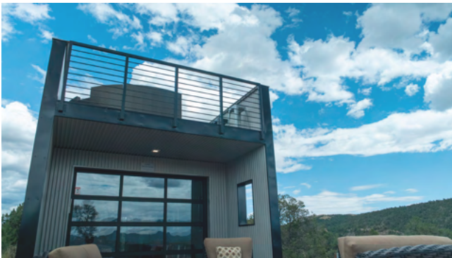
BAD ASS GARAGE View of entry with rooftop deck
